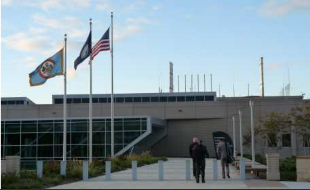
Figure 7: McConnell Public Safety and Transportation Operations Center
