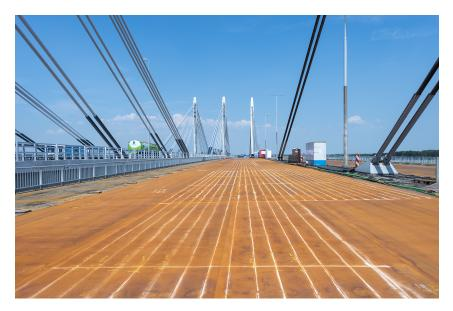
Figure 2.5: Road surface replacement during the renovation of the A50 Ewijk Valbrug in 2013 (*Credits: Thea van den Heuvel* - *Rijkswaterstaat Image Bank*)
