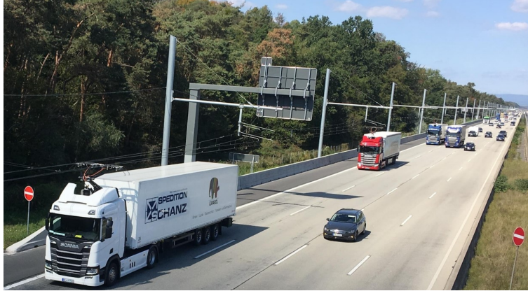
Figure 5.7: Infrastructure preview of overhead conductive technology (photo from Siemens)
