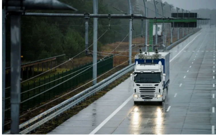
Figure 1.2: Overhead conductive ERS (Muelaner, 2020)
