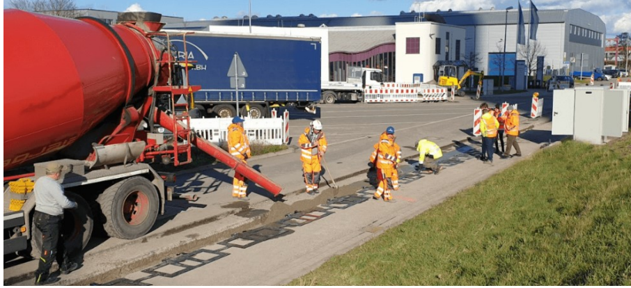
Figure 5.11: Pavement construction (photo from Electreon)
