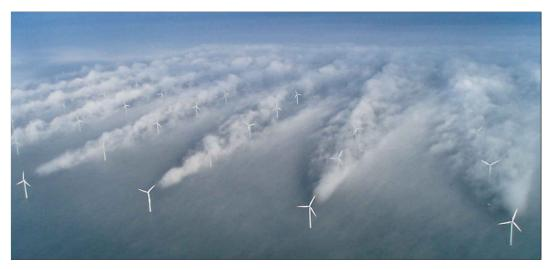
**Figure 1-1:** The Horns Rev offshore wind farm near Denmark under foggy weather conditions. The flow wakes formed by turbines extracting energy from the wind are clearly visible. [10]
