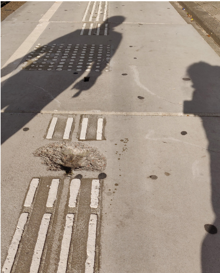
FIGURE 15-3 Damaged concrete flooring at a temporary stop.
