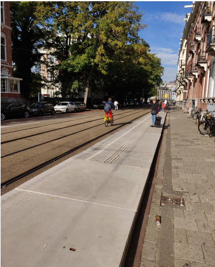
FIGURE 2-4 No tactile lines at a segment of the temporary stop.
