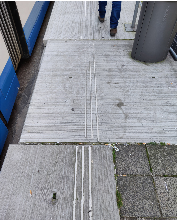
FIGURE 15-6 Uneven concrete flooring at a temporary stop.
