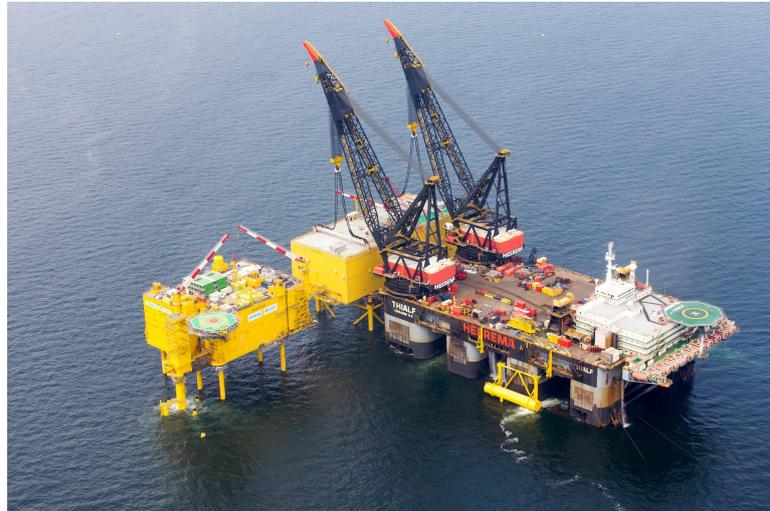
Figure 3.1: Offshore wind power converter station installation on a jacket by the HMC Thialf (HMC, 2015)
