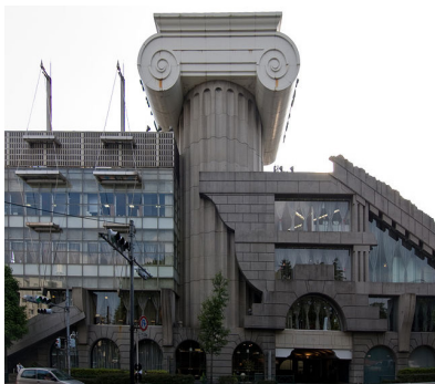
O M2 Building. Photograph by Wiiii, May 27, 2008. Wikimedia Commons.
