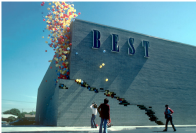
E BEST Notch Building . Photographer unknown, 1977. SITE.
