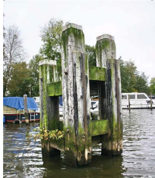
Figure 1: Mooring pole Zwartsluis/Netherlands
