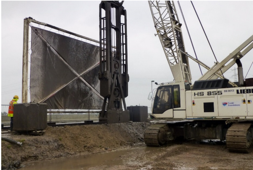
Figure 14: Installation of a concrete diaphragm wall near the outer edge of the embankment crest with a grab trenching machine, near Schoonhovenseveer, Netherlands.
