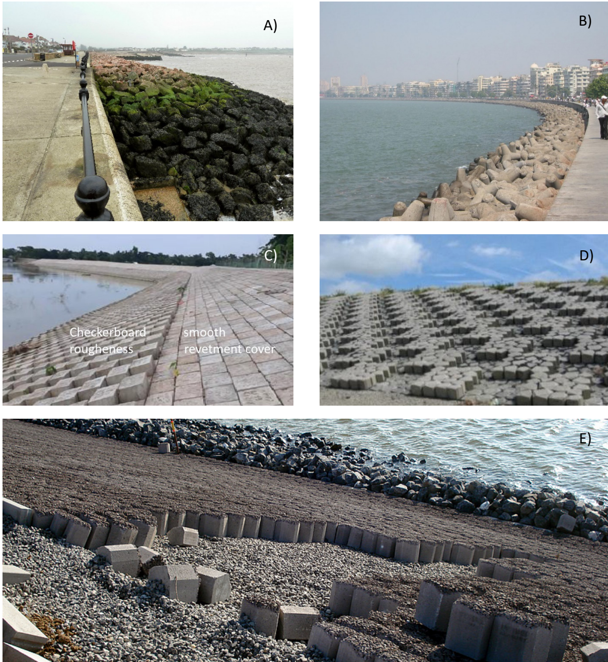
Figure 8: High-roughness revetments. A) Rock armour revetment in Hampton-on-Sea, England (photo by Storve book , CC BY licence). B) A revetment from concrete tetrapod elements in Mumbai (photo by Kelisi , CC BY SA licence). C) A revetment with checkerboard roughness pattern at the Padma river in Bangladesh (adapted from Asaduzzaman; Wang, 2020). D) Checkerboard roughness created with concrete Basalton columns at the Hondsbossche Zeewering, The Netherlands (Jonkman et al., 2021). E) Erosion protection on the outer slope of a river embankment under construction near Ammerstol, Netherlands.
