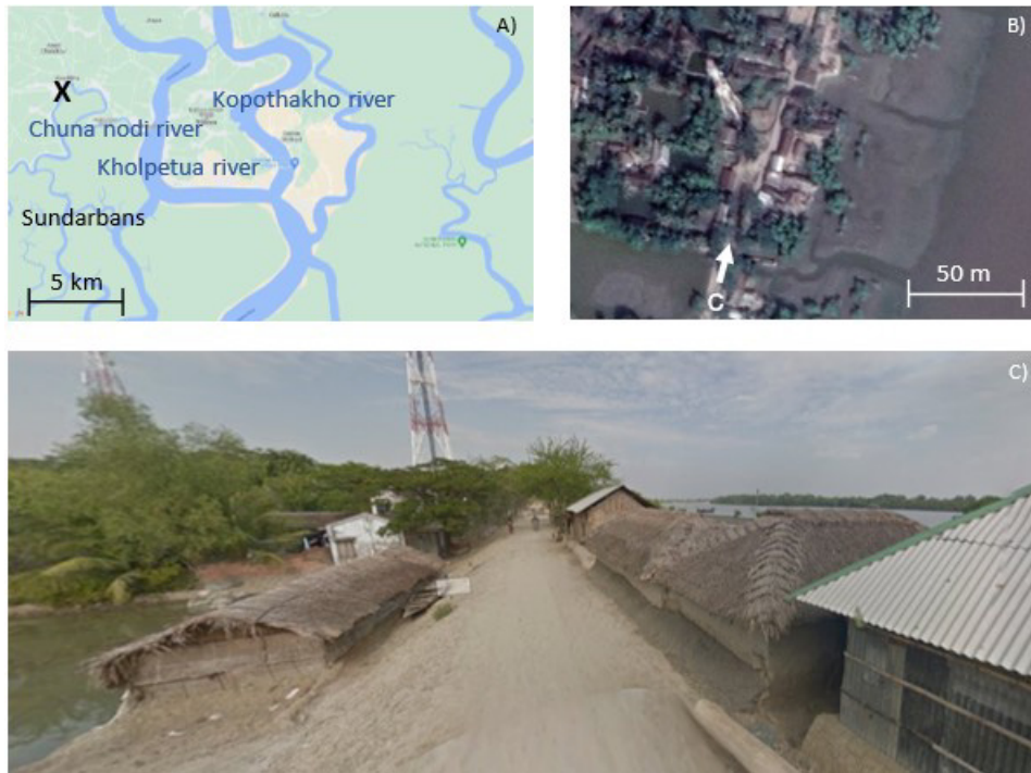
Figure 5 A) The location of the embankment site (marked by the 'X'). B) An aerial photo of the site. Letter C indicate where the photos in panel C is taken, with the arrow for the view direction. C) Photo of the embankment (gravel road), with buildings at both sides. Water at the left of the road is an aquaculture pond, at the top right is the river. Sources: Google Maps; Google Earth, CNES, Airbus, Maxar Technologies; Google Streetview.
