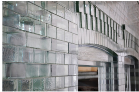
Fig. 1 View of the Crystal Houses, assembled from cast glass elements mimicking ceramic masonry. Derived from (Oikonomopoulou 2019)
