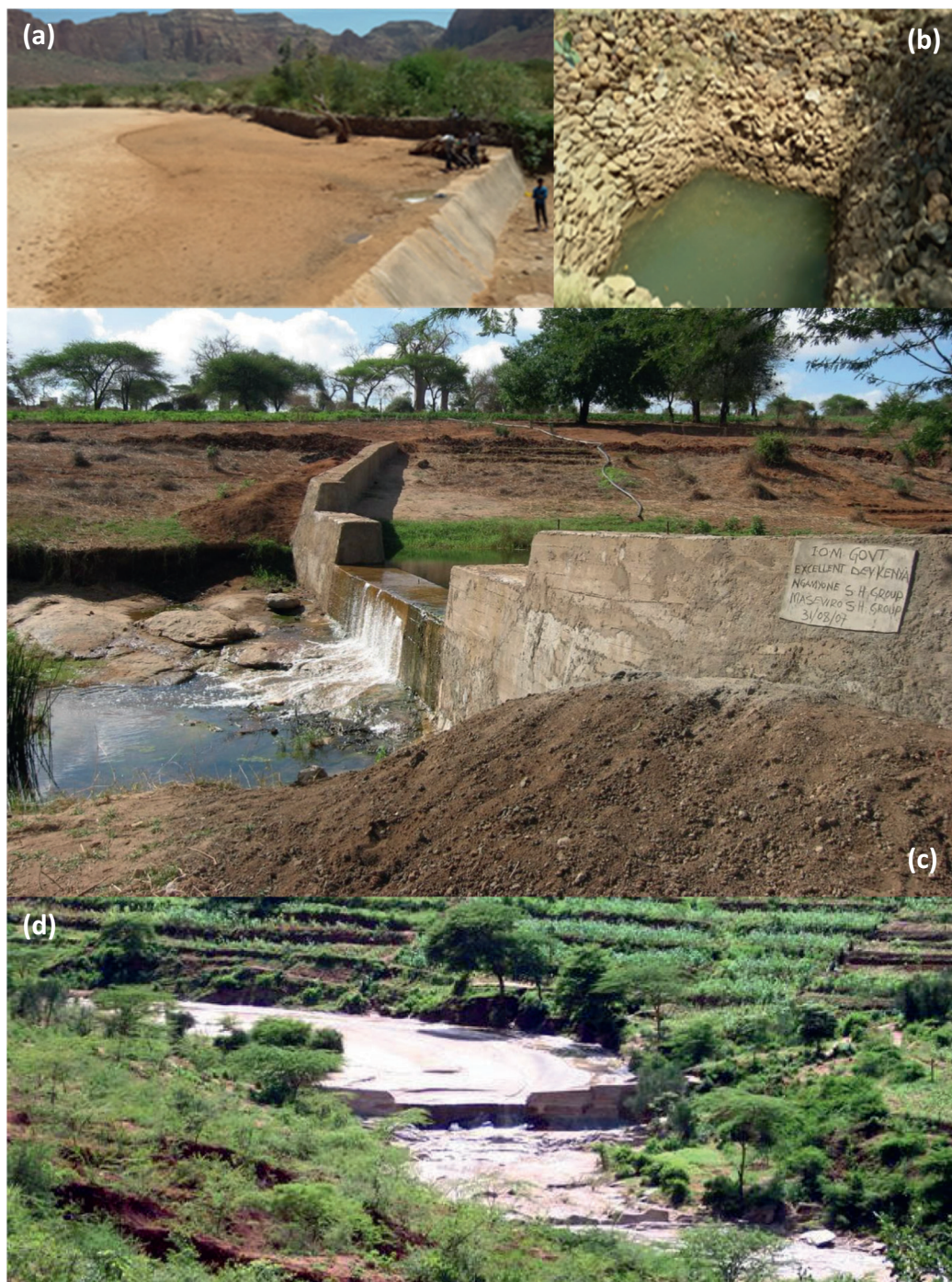
Fig. 2. Pictures of sand dams: (a) sand dam in May Gobo (Ethiopia) and scoop holes (b); (c), (d) sand dams in Kenya. Sources: (a) and (b) – photo -by Lorenzo Villani; (c) and (d) Excellent Development - (CC BY-NC-ND 2.0).
