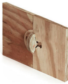
Slot connection (DeArchitect, 2013)
