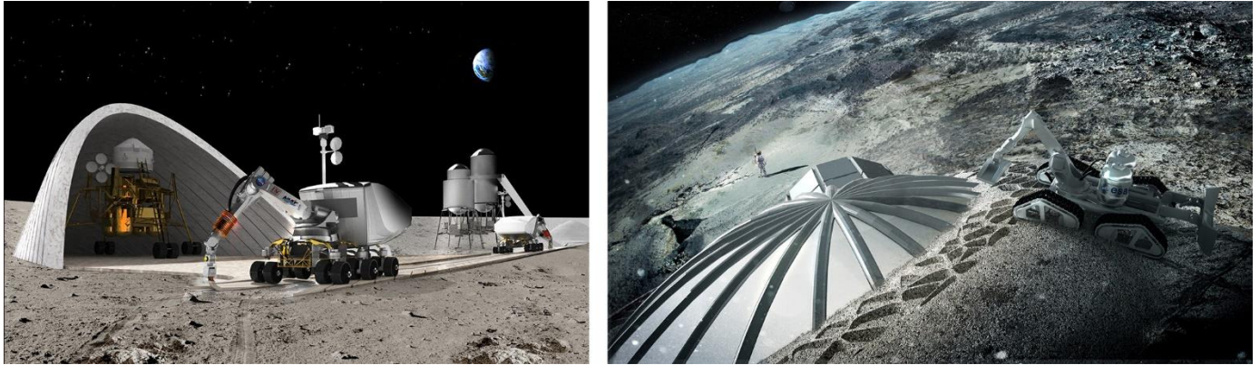
Figure 3: Left - A Contour Crafting robot prints a road in front of a hangar for a lunar lander, Source: Behnaz Farahi/NASA, Right - 3D printing concept for lunar based using in situ resources, Source: Foster + Partners
