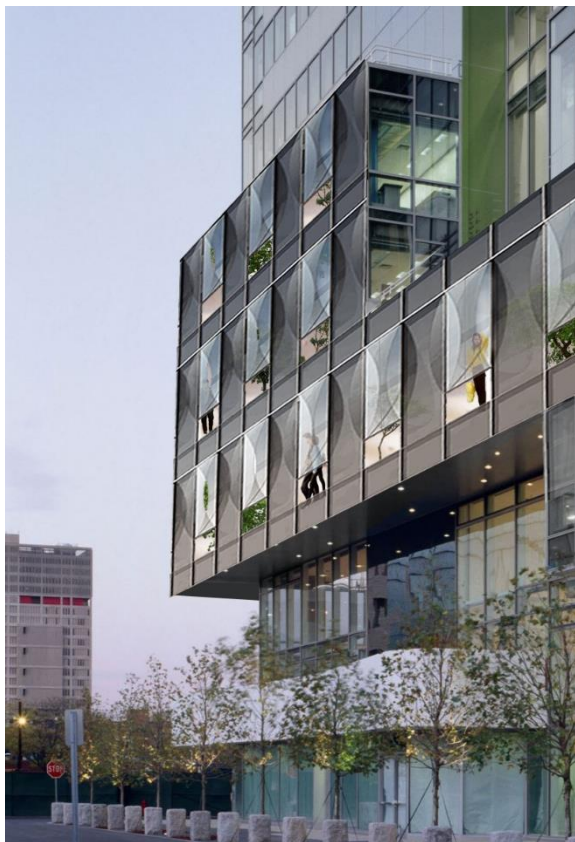
Current situation of the outside windows vs. proposed situation of exterior windows
