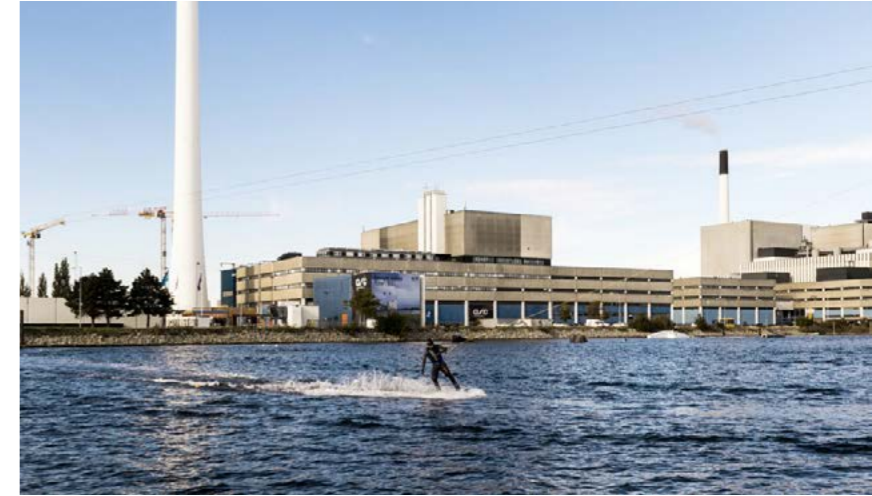
INCINERATION PLANT 1, DENMARK NOT GIVEN
