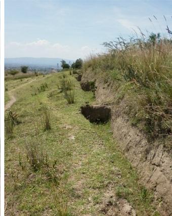
*Fig. 2.3.5. Trenches constructed perpendicular to the water flow.*
