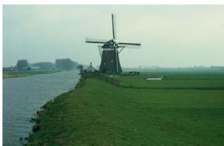
Figure 1. Regional flood defence in the Netherlands (Rijkswaterstaat)
