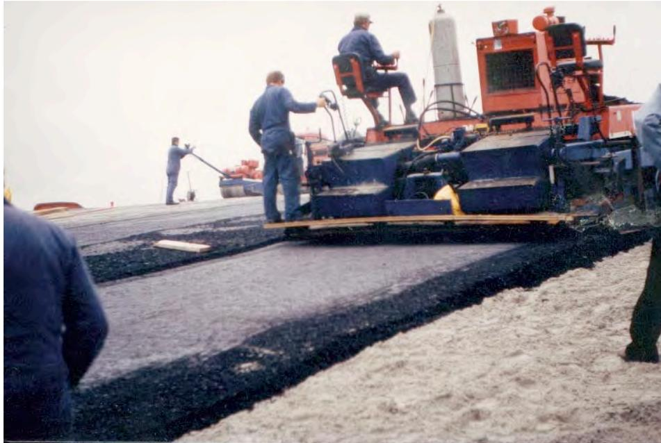
Figure 13-22 Construction of an asphalt revetment (photo Netherlands Pavement Consultants)
