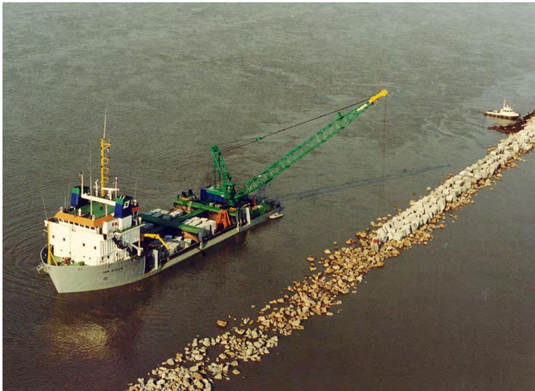
Figure 13-24 Placing elements on a breakwater with crane ship (van Oord)
