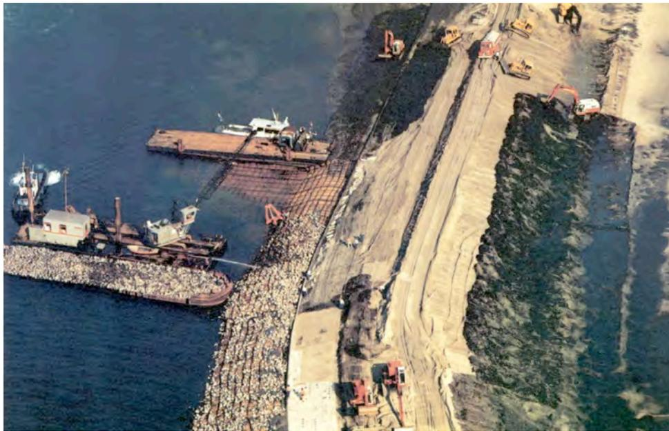
Figure 13-16 Placing fascine mattress on revetment
