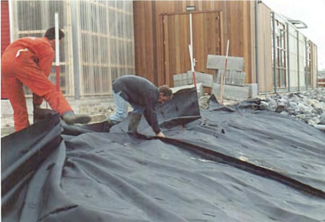
Figure 13-11 Placing geotextile in simple revetment (Johan van der Ham)
