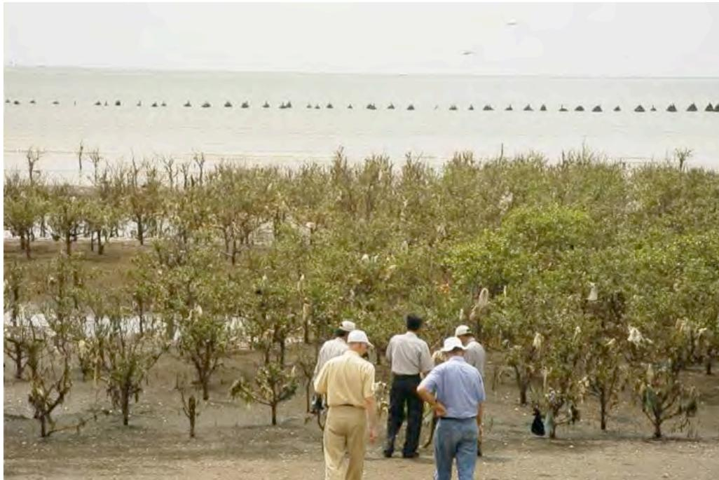
Figure 12-20 Mangrove reforestation with wave load reductor
