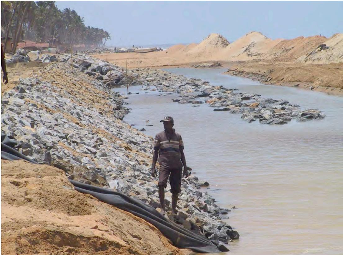
Erosion protection in Sri Lanka (photo Pilarczyk)
