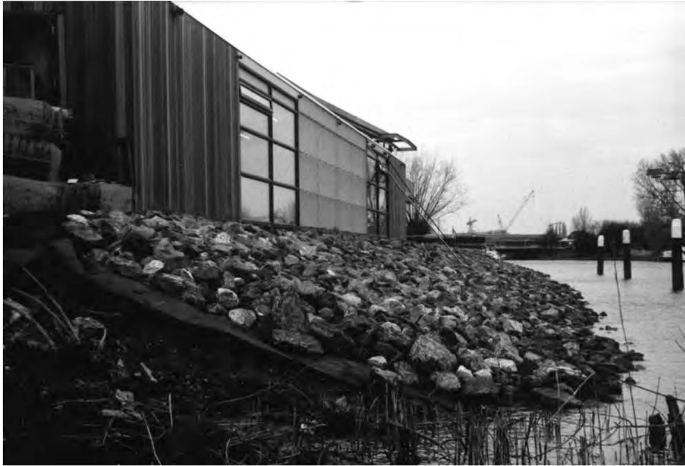
Figure 11-16 Simple bank protection with geotextile
