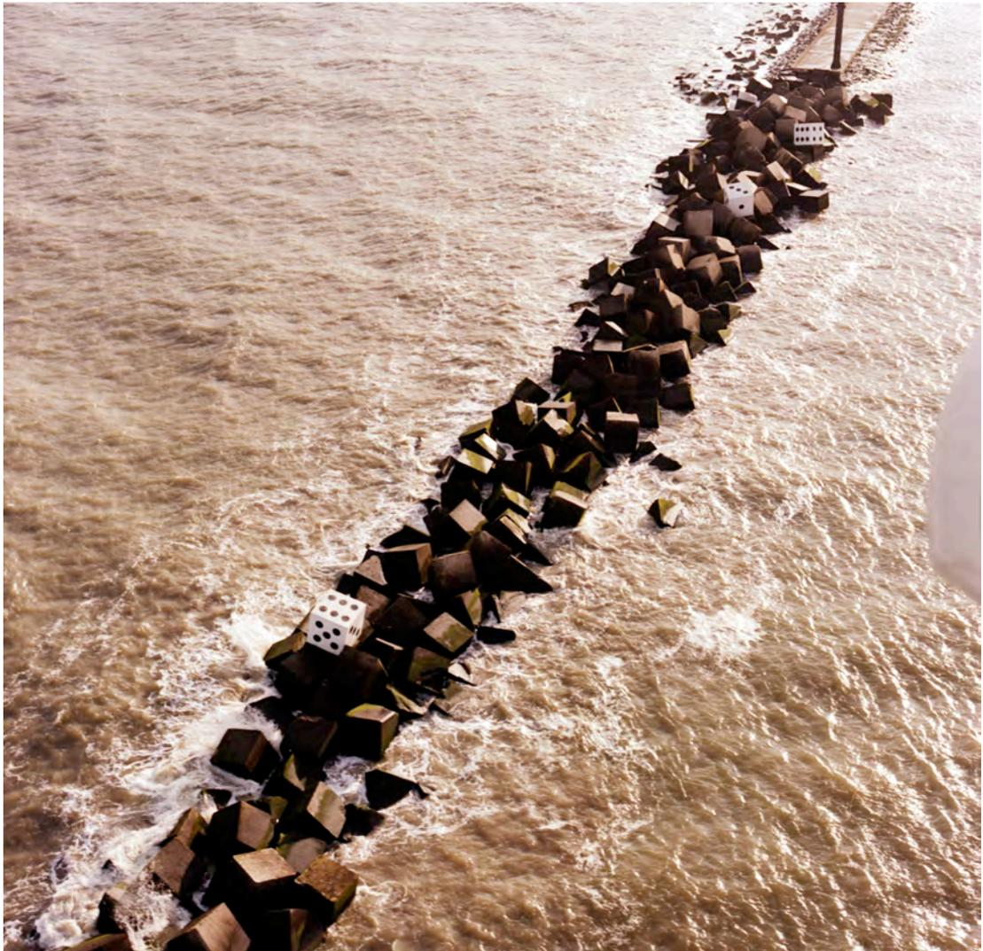
Dice block on the breakwater of Hook of Holland
