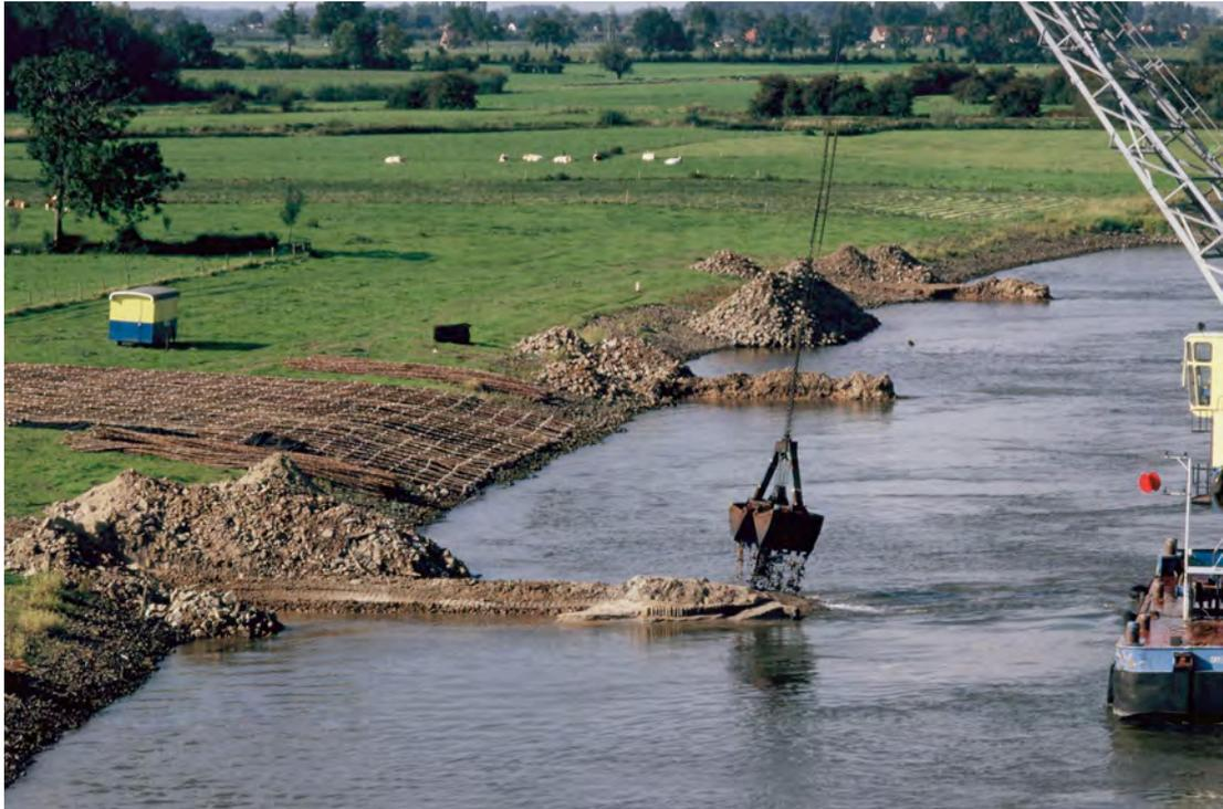
Figure 13-19 Construction of a river groyne (photo Rijkswaterstaat)
