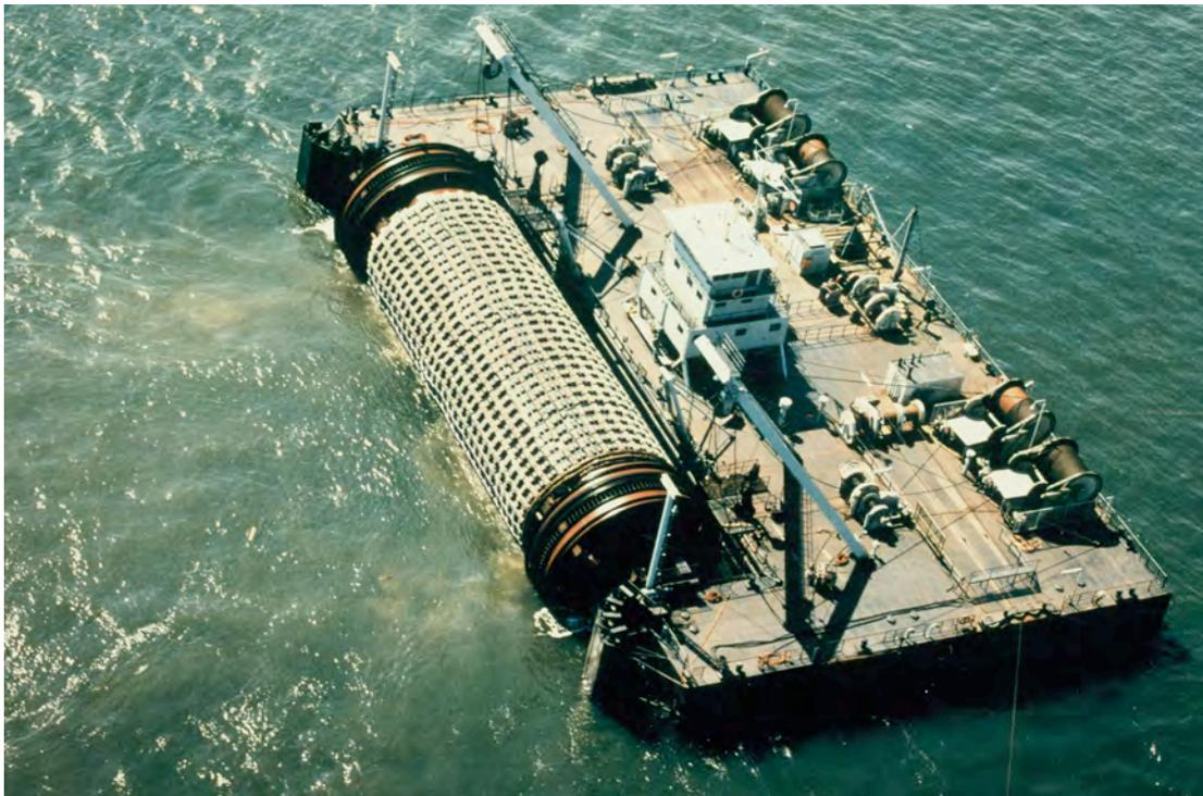
Figure 13-10 Sinking block mat in Eastern Scheldt (Rijkswaterstaat)
