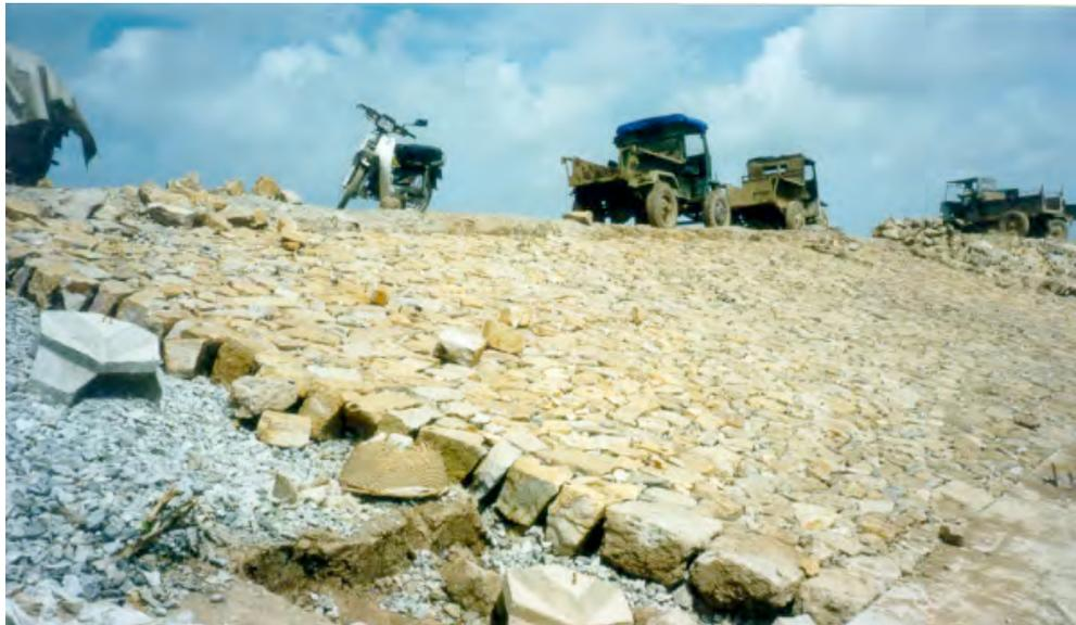
Figure 11-24 Placed block revetment (Vietnam, photo Verhagen)
