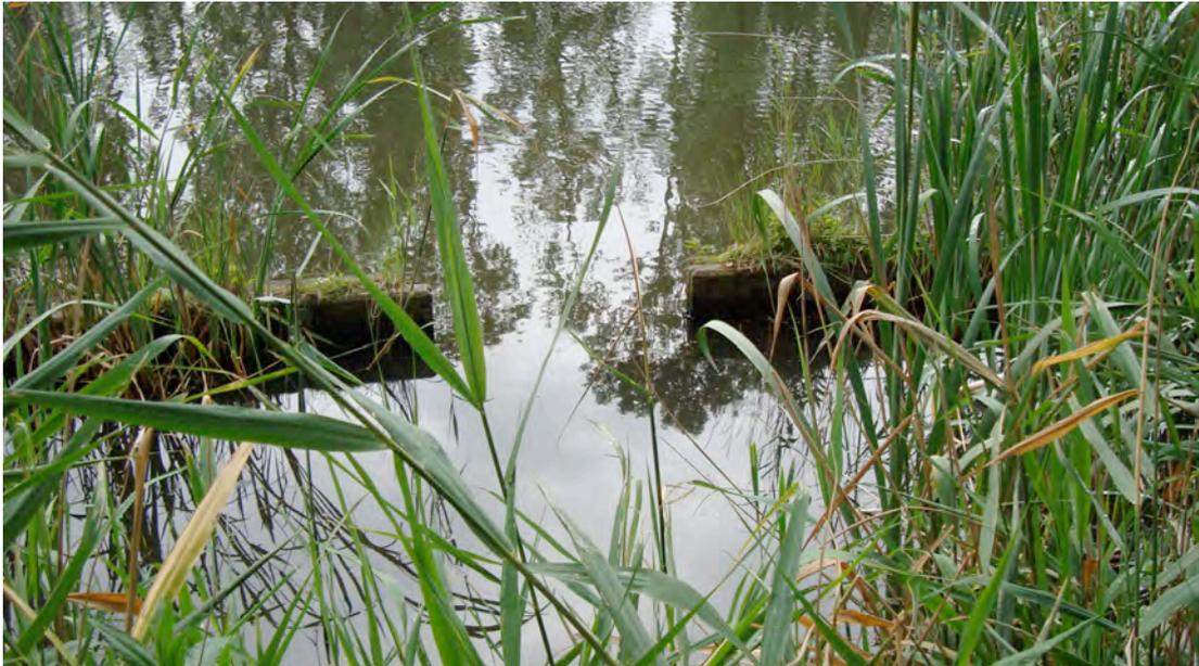
Figure 12-5 Gap in a sheetpile, in this case especially to allow beavers to cross the sheetpile (photo Verhagen)
