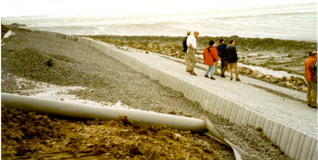
(Granular filter and a geotextile under a Hydroblock revetment, photo H.J. Verhagen)
