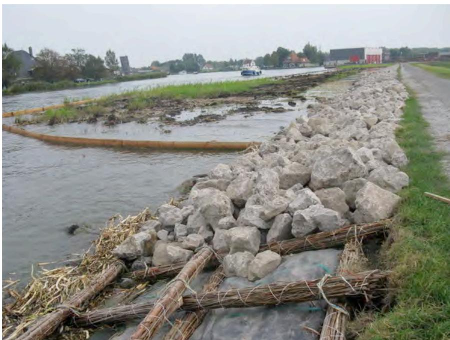
Figure 11-8 Geotextile under mattress (photo Griendhouthandel)
