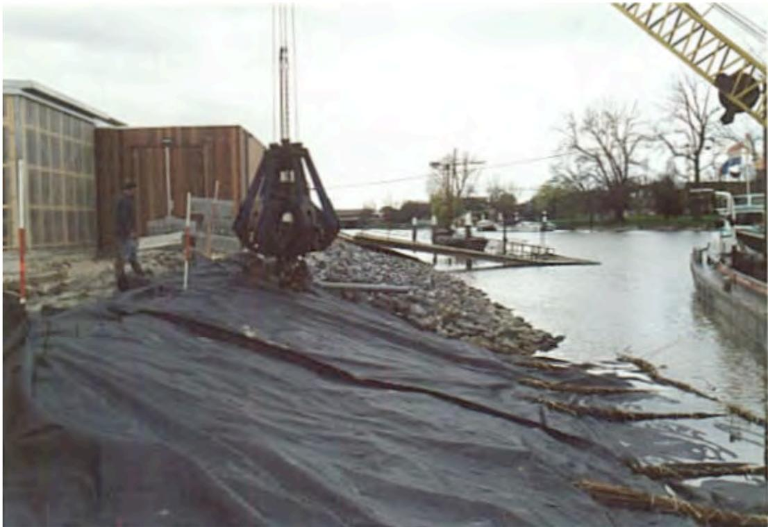
Figure 13-13 Placing stones with floating crane and grab (Johan van der Ham)
