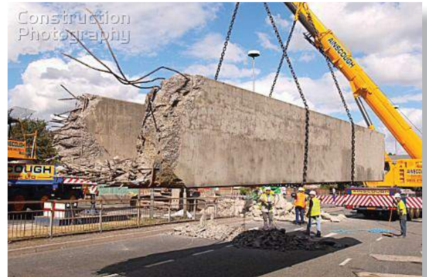
Figure 17: Lifting of a section of a footbridge [37]
