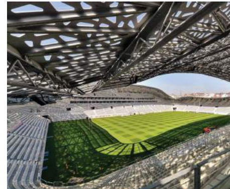
Figure 4: UHPFRC application in Jean Bouin Stadium. [10]
