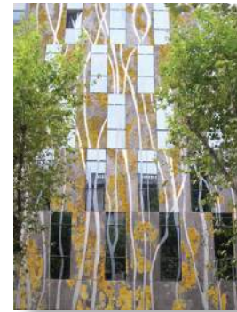
Figure 12: Simulation of the vegetated facade, at the Ako suits hotel in Barcelona.
