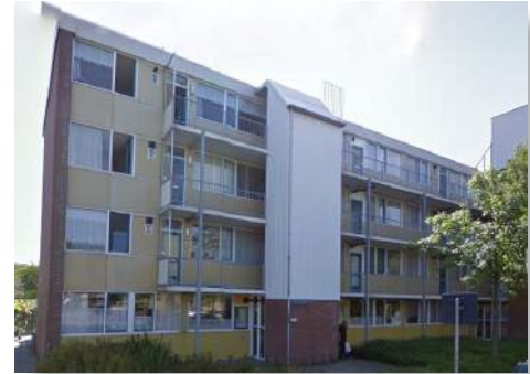
Figure 18: Reuse of concrete elements in residential buildings Vrijheidstraat. [38]
