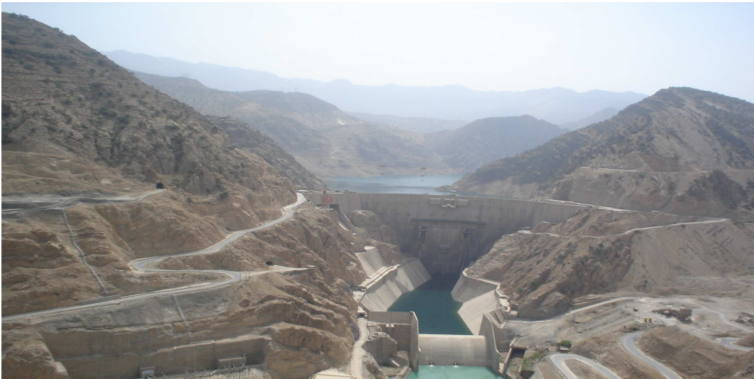
Figure 1-5. Karun III arch dam in Iran, H = 205\text{ m} , maximum discharge capacity of 18000\text{ m}^3/\text{s} through chute and overfall spillways and orifices (IWPCO, 2006).
