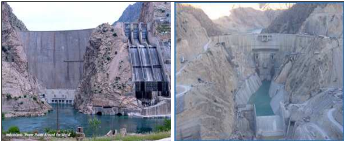
Figure 4-1. Plunge pool on Karun Dam in Iran (IWPCO, 2006)
