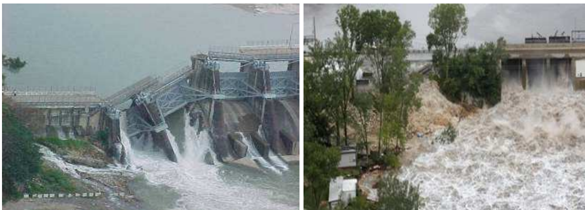
Figure 1-12. Dam break in the Shih-Kang Dam Taiwan, 1999 (left) [5]. Catastrophic dam-break flow in Delhi Dam, Maquoketa River, Iowa, United State, 2010 (right) [6].
