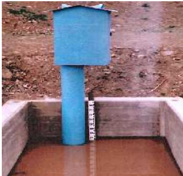
Figure. App 2.2. Automatic streamgage on Ziaran channel
