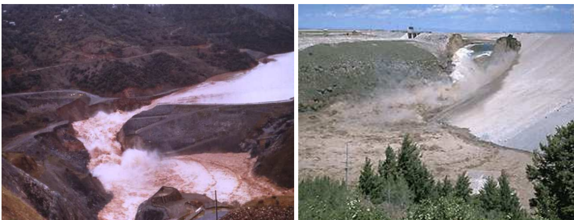
Figure 1-13. Failure of the Auburn Cofferdam on the American River, 1986 (left) [7]. Teton Dam collapse, Idaho, United States, 1976 (right) [8].
