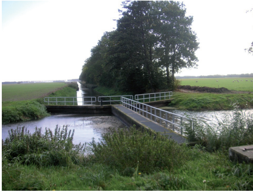
Figure 7-11 Aqueduct in the Noordoost Polder; a concrete water supply channel crosses a water discharge channel (source: Zuiderzeeland Water Board).
