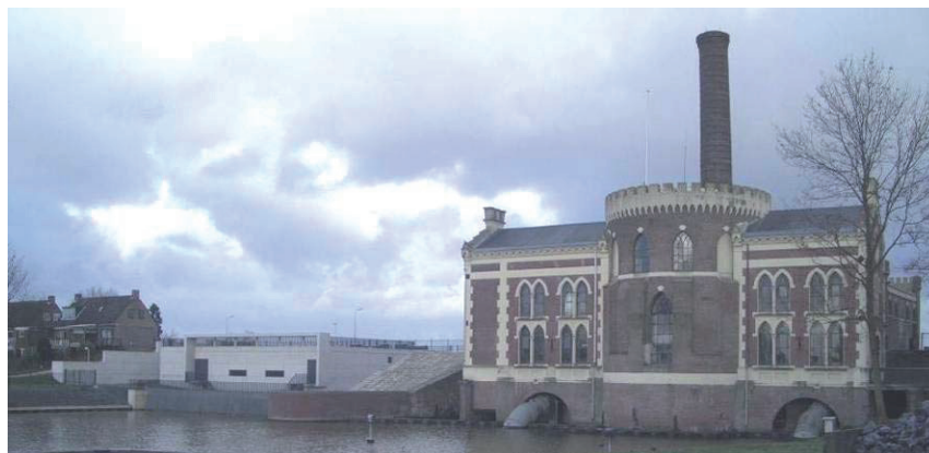
Figure 3-1 The new ( 1,275 \text{ m}^3/\text{min} ) and old ( 819 \text{ m}^3/\text{min} ) pumping stations at Lijnden in the north of the Haarlemmermeer polder.
