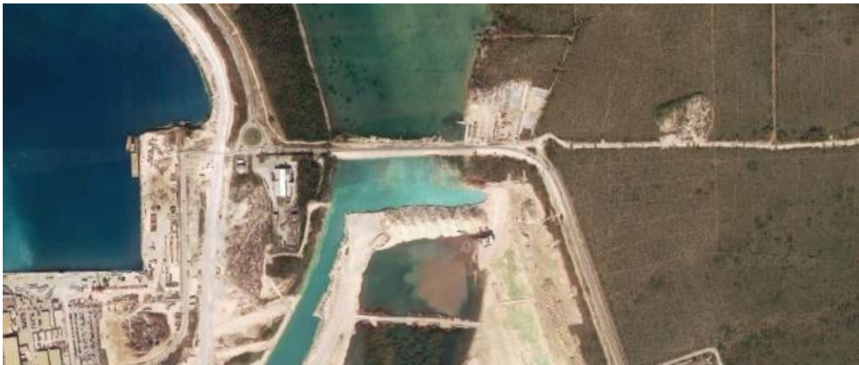
Fig 132: Existing bridge on the northern harbor area, zoom in on figure 131.(source Googlemaps 2020)
