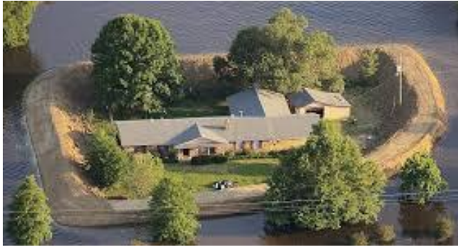
Fig 42: Individual protection measure
