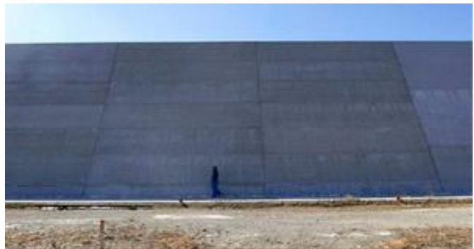
Fig 45: No view on the ocean due to the structure separating and disconnecting certain areas.
