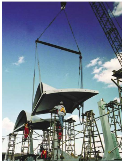
Fig.Ap3.3. Crane set of canopy [Courtesy of Tucker Photo]
