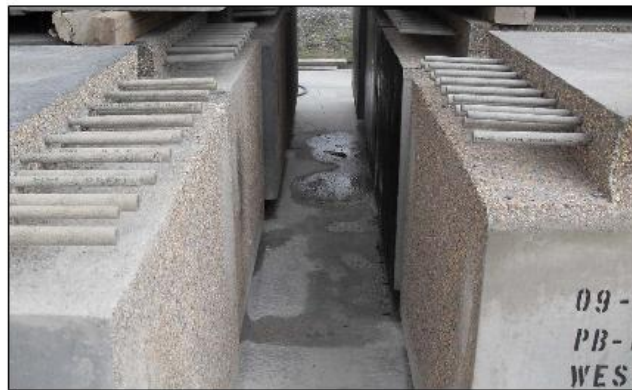
Fig.Ap3.35. End of box girders showing reinforcing and exposed aggregate roughening to enhance
