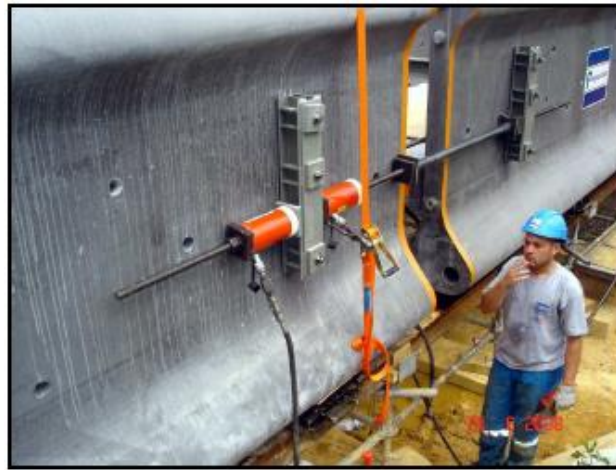
Fig.Ap3.11. View of the interim clamping system
