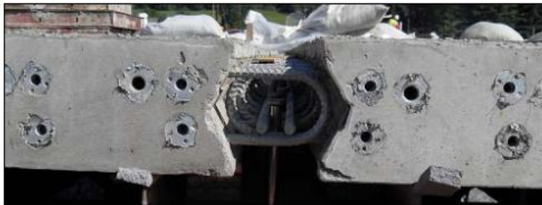
Fig.Ap3.31. End view of the UHPC joint fill between precast deck panels at the abutment
