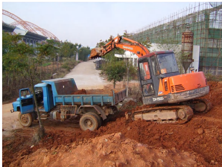
Figure 20 Excavator and Truck in the delivery
