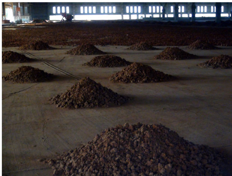
Figure 21 Soil paved in the experiment hall
