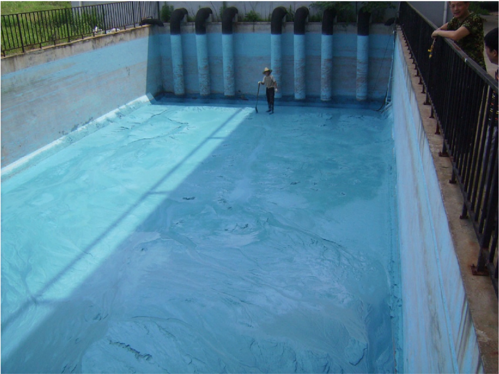
Figure 6 Sediment Basin and Reservoir
