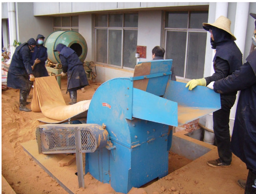
Figure 23 Grinder to reproduce the soil
