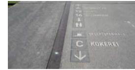
Cycling lane Width:3-4m Asphalt with signs
