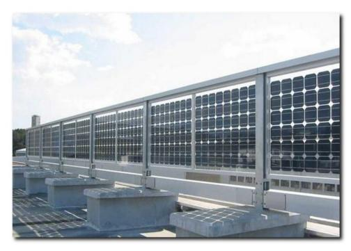
Figure 8.15: Vertically mounted bifacial PV modules [18].
