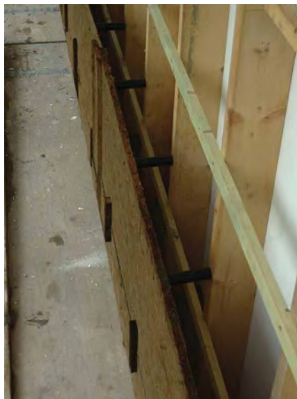
Fig.5: Exposed frame internally for permanent shuttering, showing horizontal rails.
