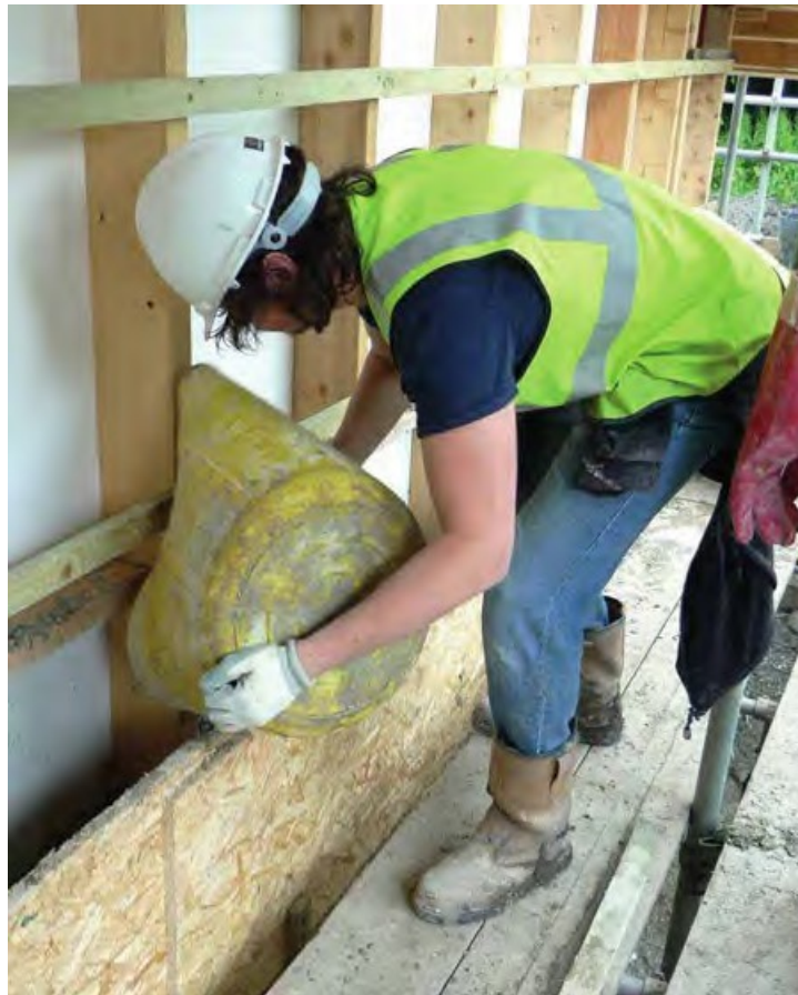
Fig.7: Placing freshly mixed hempcrete into shuttering (William Stanwix & Alex Sparrow)
