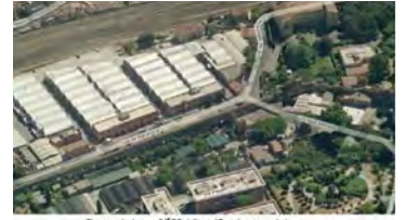
The aqueduct as an edge defines different program, below we see industrial area and residential area
