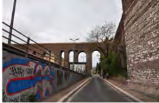
We see the spatial phenomenon of crossing between the aqueduct and a road
