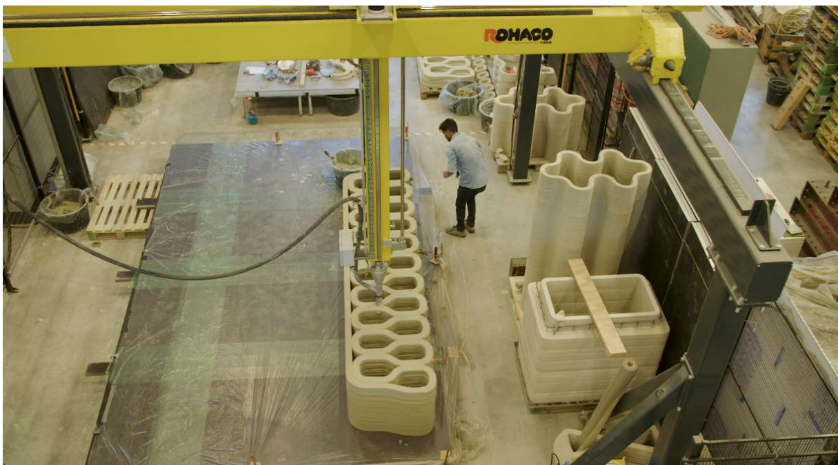
Figure 15: The robotic 3D concrete printer. Reprinted from: 3Dprintedhouse (2018).
