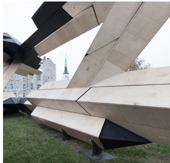
Figure 107: Close-up of assembled components under a 45 degree angle. Adapted from: Retsin (2017).
