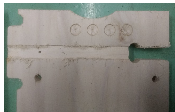
Figure 151: Photo of the right vertical beam of section four, which has splintering, or tearing, at the groove.
