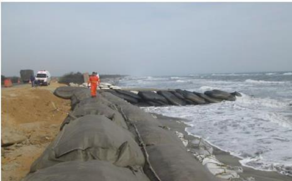
Figure 71: Photograph during construction (Sisco Ingeniería, 2015)
