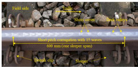
**Fig. 1.** Short pitch corrugation with a wavelength of about 40 mm in the Dutch railway network. Corrugation wavelength refers to the distance between two adjacent shiny crests. This corrugation is developed on a straight ballasted track with duo-block sleepers and fastenings with the Deenick clip. Less severe corrugation is found on the other rail at the same site.
