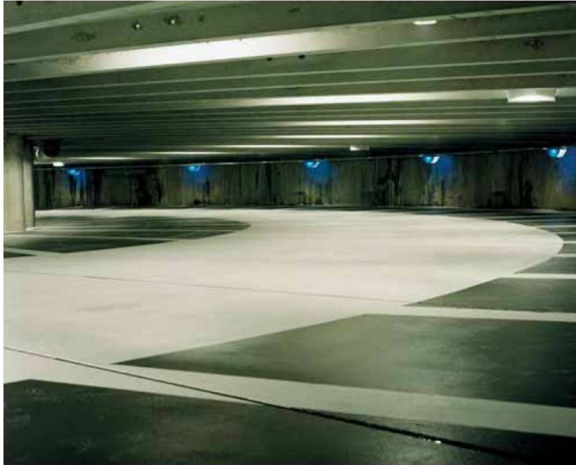
Figure 6: parking garage Ossemarkt Groningen
