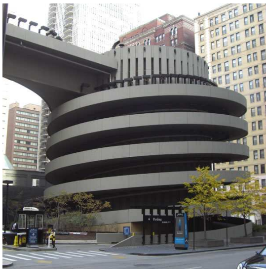
Figure 7: example of a helical ramp at hancock garage
