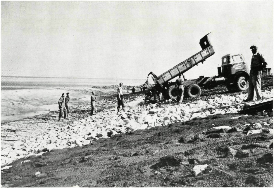
Stone revetment grouted with mastic asphalt in the tidal zone.
