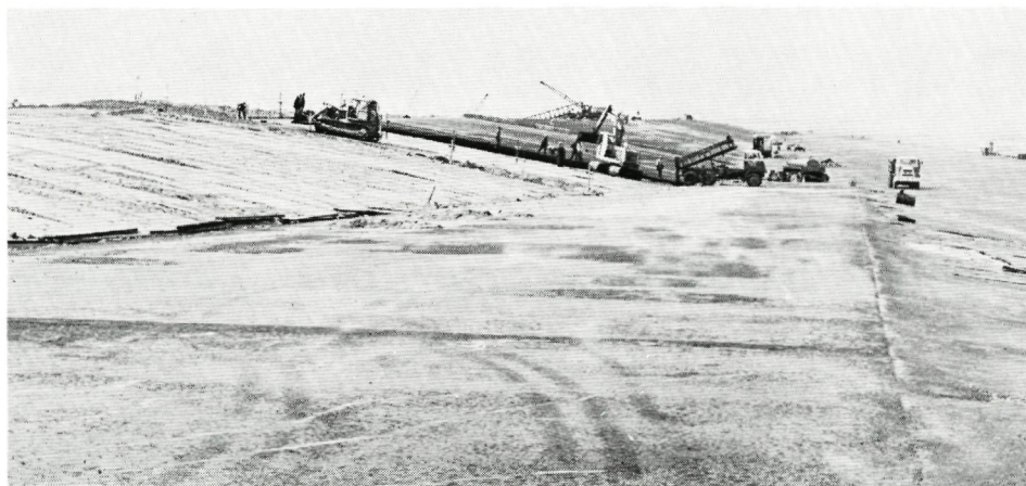
Berm and 1 : 6 slope gradient on the Brouwersdam.
