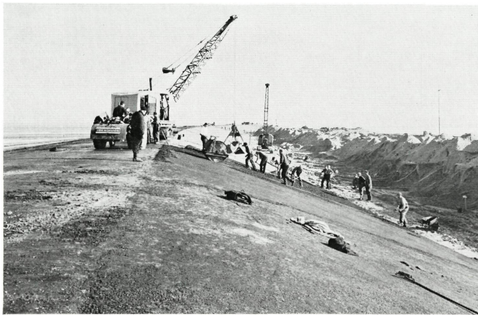
Asphalt compaction on a slope with a gradient of 1 : 3 on the Brouwersdam.
