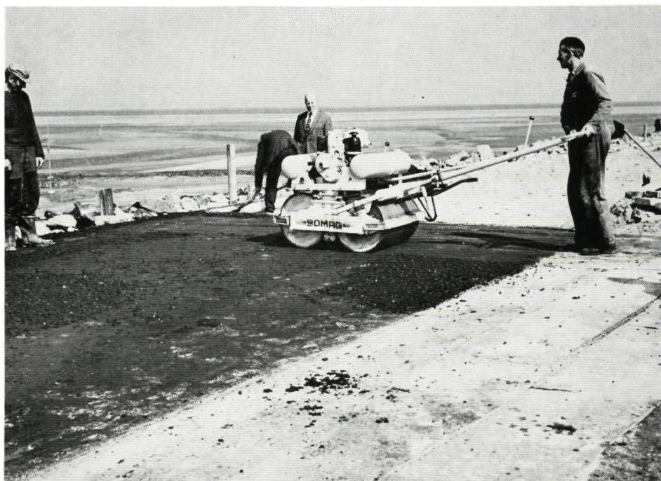
Compaction of a asphalt revetment on a berm.
