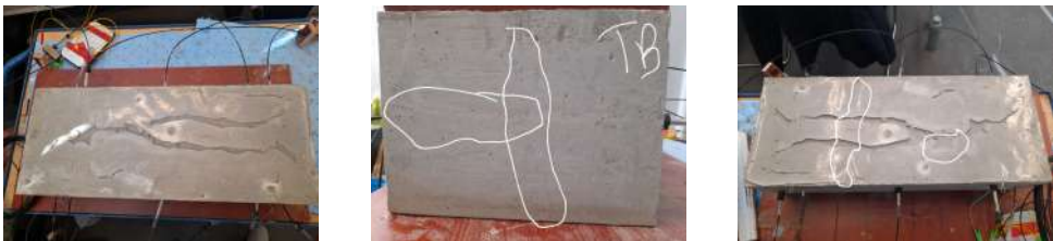
Figure 6.1: Cracks developed on concrete surface after curing
