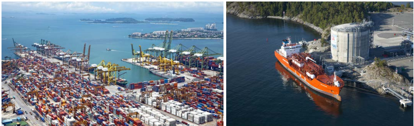
Figure 1.12: Left: Container terminal (by pxhere.com is licenced under CC0 1.0); right: LNG-terminal (by Jan Arrhénborg / AGA is licenced under CC BY-SA 3.0).
