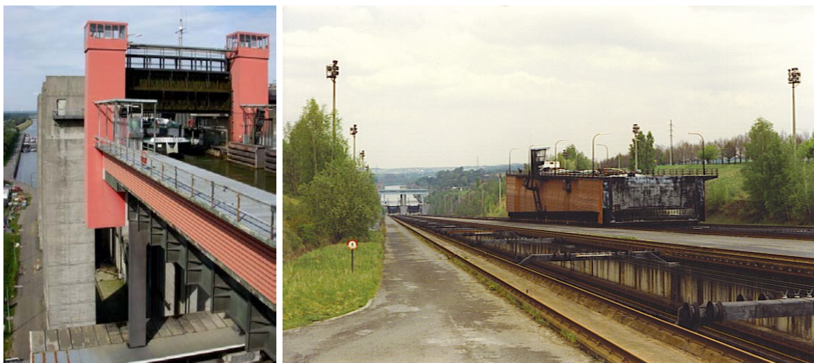
Figure 1.24: Left: Ship lift at Scharnebeck, Germany (by Holger Ellgaard is licenced under CC BY-SA 3.0); right: Inclined slope of Ronquies, Belgium (by Jean-Pol Grandmont is licenced under CC BY-SA 3.0).
