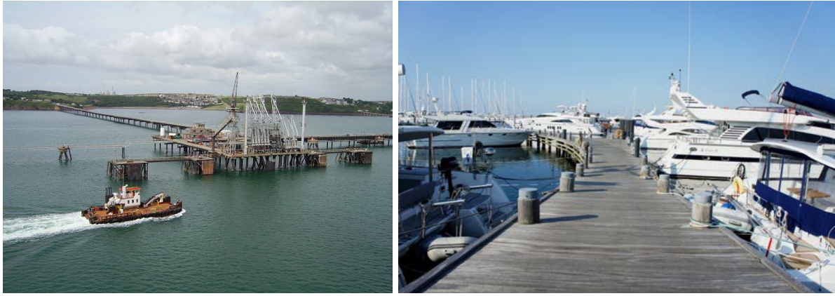
Figure 1.20: Left: Oil jetty, Total refinery, Milford Haven (by Richard Webb is licenced under CC BY-SA 2.0); right: Marina jetty (by pxhere.com is licenced under CC0 1.0).
