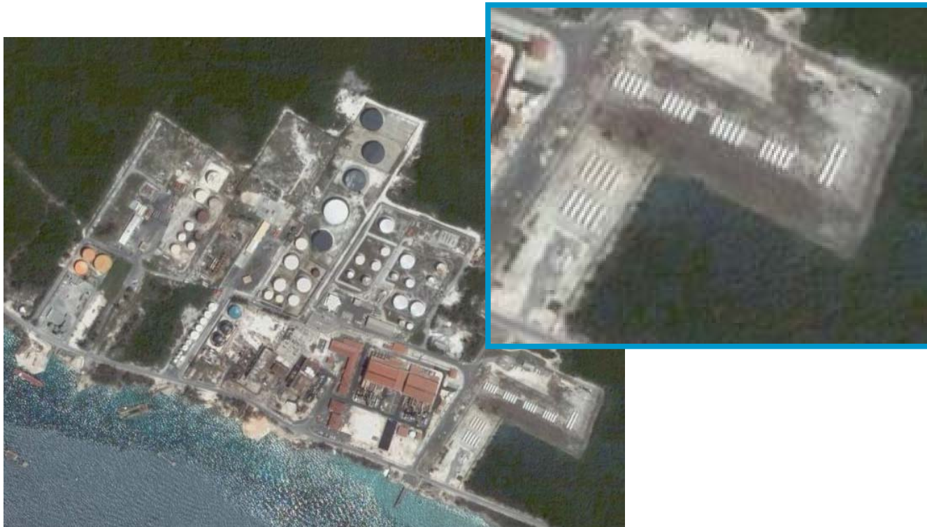
Figure 6-3: Detailed view of LPG storage area at current Power Plant
