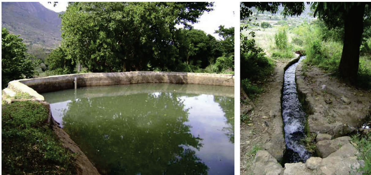
Figure 2.2: Manoo irrigation system, including the micro-dam and canal (Kemerink et al., 2007).
