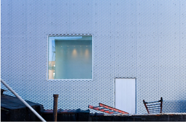
opening on north elevation
