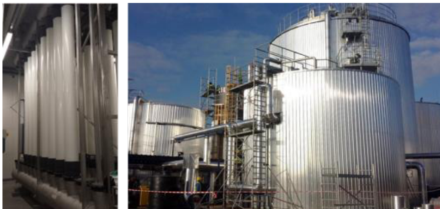
Figure 1.2 Industrial AnMBR (Memthane®, courtesy Biothane) at a food company; left: external crossflow membrane skid, right: anaerobic mixed tank bioreactor.
