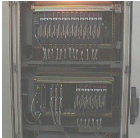
Figure 4.17 Programmable Logical Controller
