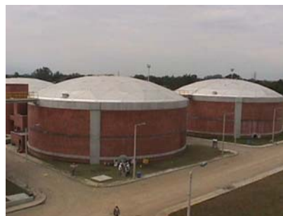
Figure 3.33 Anaerobic digesters
