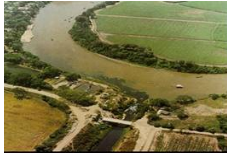
Figure 3.10 South Channel discharge point to Cauca river
