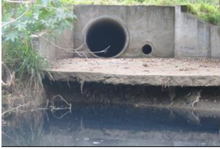
Figure 3.12 Collector Margen Izquierda discharge point, before collapsing in 2003.
