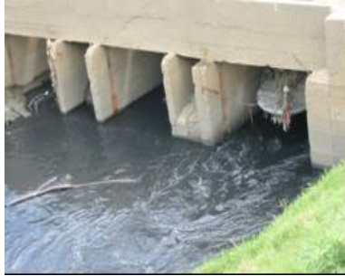
Figure 3.17 Exit channel from Paso del Comercio pumping station
