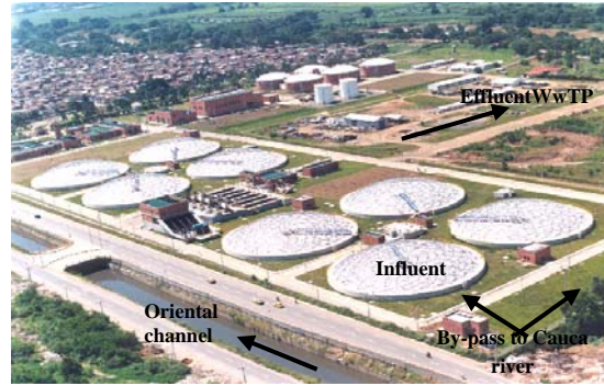
Figure 3.25 General scheme Cañaveralejo wastewater treatment plant (C-WwTP)
