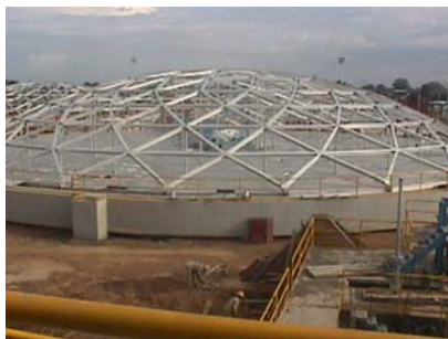
Figure 3.29 Primary sedimentation tanks
