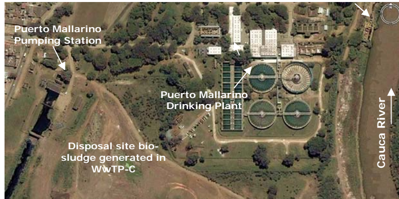
Figure 3.35 Location final disposal site for the bio-sludge coming from C-WwTP
