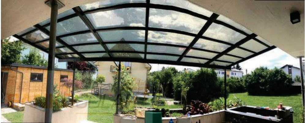
Figure 1.2: A glass patio cover based on highly transparent Cadmium Telluride thin film solar cells. [27]
