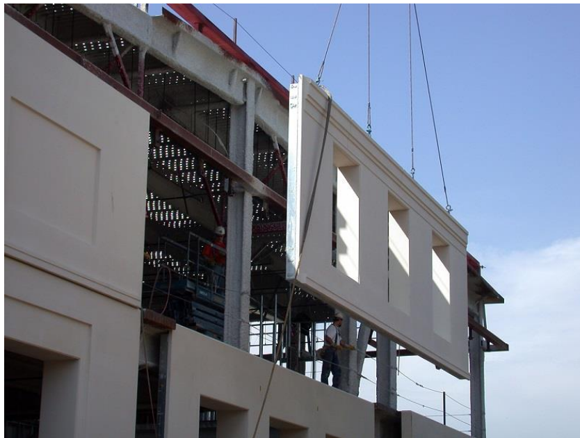
Figure 15: Installation of a precast concrete panel (Mishra, 2020)
