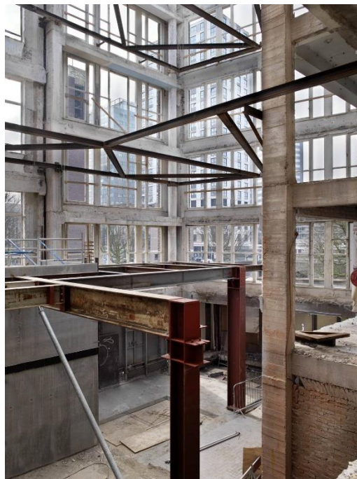
Figure 4: Interior of Hoogstraat 168-172 with the Donor Skeleton clearly visible (IMd Raadgevende Ingenieurs, 2020)
