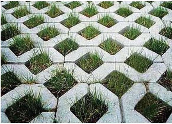
Fig. 8.16: Permeable pavers Source: http://lateameffort.blogspot.com/2010/04/road-less-traveled-pervious-pavement.html
