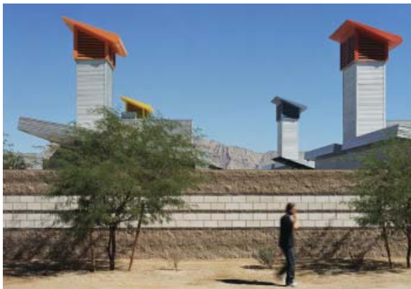
Fig. 6.23: Wind catch towers Source: buildinggreen.com
