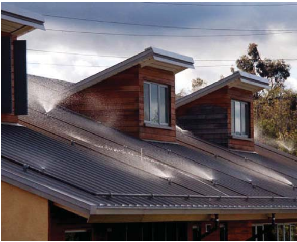
Fig. 6.20: Sprinkled roof Source: Carnegie Institute for Global Ecology
