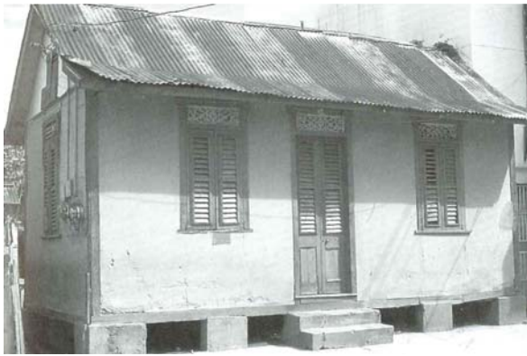
Fig. 7.8: Small house with shutters and lifted from the ground, Trinidad Source: Crain, 1994, pp. 65
