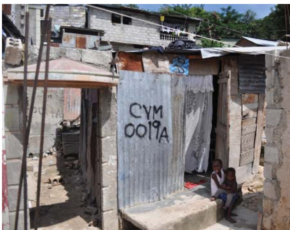
Fig. 5.20: The CRS house, Villa Rosa, Port-au-Prince Source: Author
