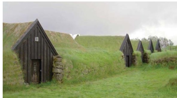
Fig. 6.29: Thermal mass by earth sheltering Source: http://coolfunclub.blogspot.com/2011/07/unique-houses-around-world.html
