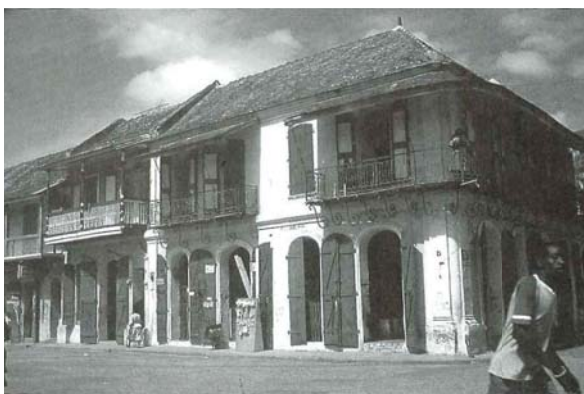
Fig. 5.16: Mixed-occupancy urban building, Cap-Haïtien Source: Crain 1994, pp. 90
