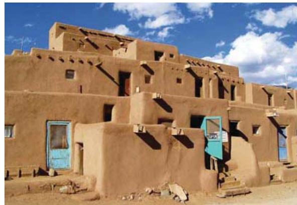
Fig. 6.30: Adobe used as thermal mass Source: http://clarkrichardson.wordpress.com/2011/11/12/the-natural-vernacular/
