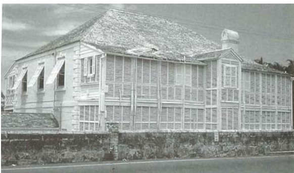
Fig. 7.6: Jacaranda residence with floor height shutters at the balcony, Bahamas Source: Crain, 1994, pp. 110
