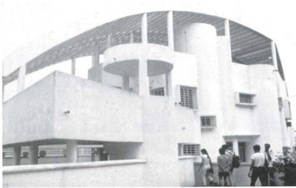
Fig. 7.16: A double roof: a shaded parasol of angled shutters. By Ken Yeang Source: Hyde, 2000, pp. 152
