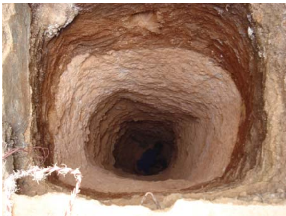
Fig. 8.11: Digging a pit for a latrine Source: Author
