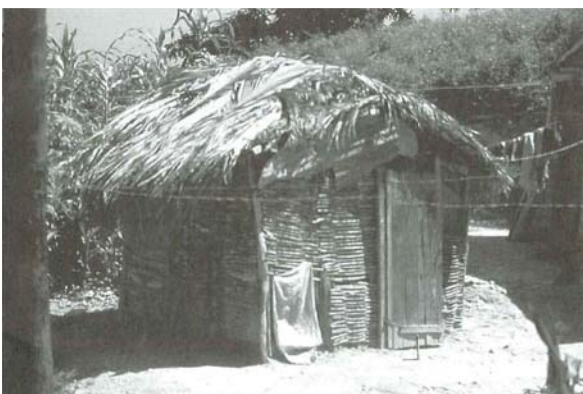
Fig. 5.13: Ajoupas or Wattle and thatch house at rural Haiti Source: Crain 1994, pp. 70
