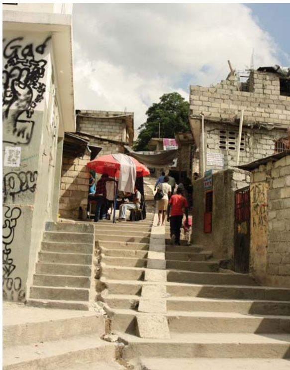
Fig. 6.13: Main street Cite Mericain with very small drainage channel and 100% paved Source: Author
