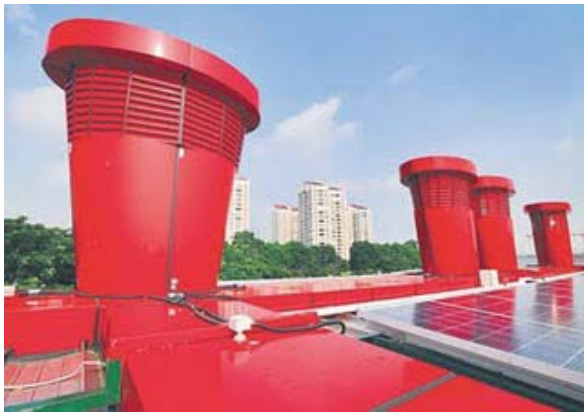
Fig. 6.22: Solar radiation heats up the solar chimney and ducts Source: http://greenbuildings-in-the-world.blogspot.com/2009/10/green-buildings-zero-energy-structure.html
