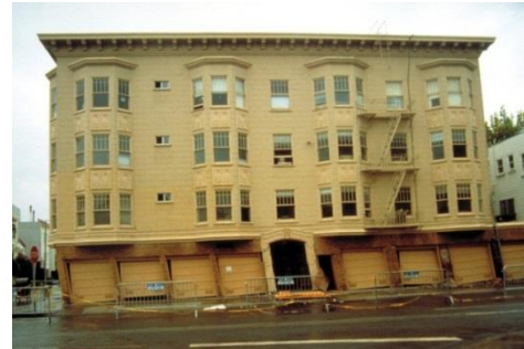
Figure 3.18: Soft ground floor collapse [images.google.nl]
