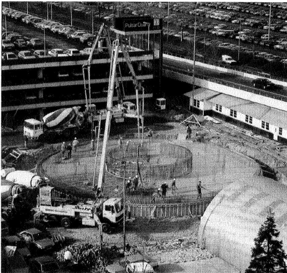
Figure 1.18: Construction foundation slab air traffic control tower Schiphol [Weersma, S., 1991]
