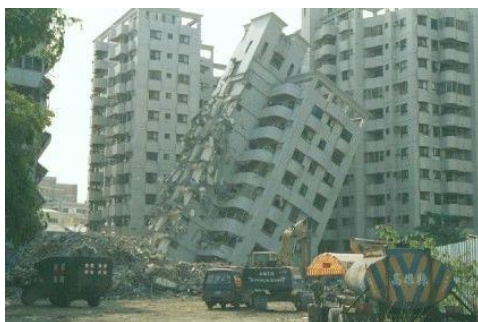
Figure 3.21: Asymmetric collapse [images.google.nl]
