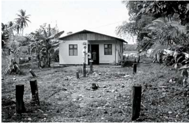
Fig. 6.14: A bamboo house that survived a 7.6 magnitude Richter scale earthquake in Costa Rica. The short poles in the foreground are remains of a timber house that could not endure the earthquake (Janssen, 2000).
