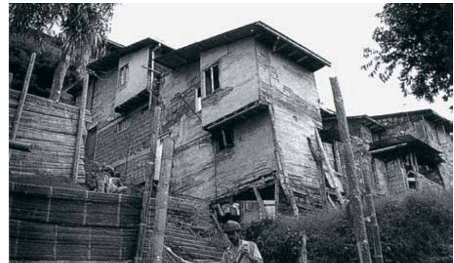
Fig. D2: Houses made of untreated bamboo (photos by Jorge A. Gutiérrez). Preservation and maintenance of bamboo houses (D1) makes them last longer than those uncared for (D2) (Liese, 2003, pp. 179).
