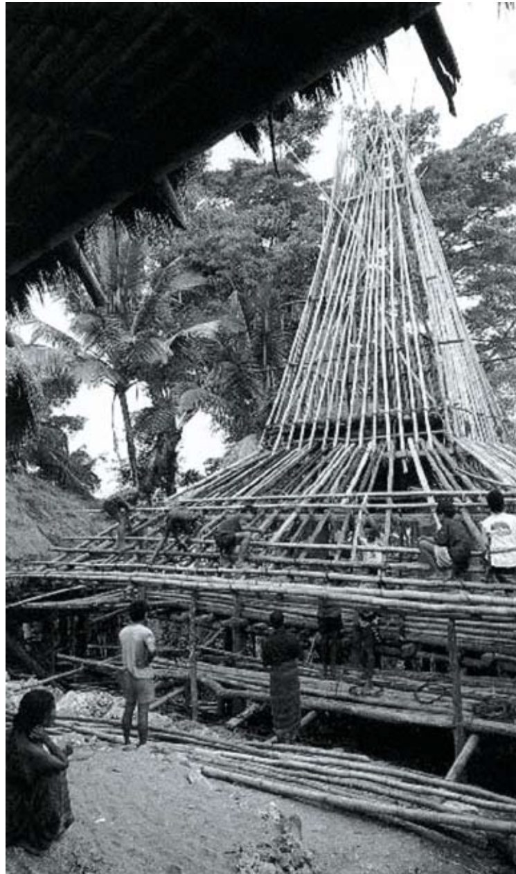
Fig. 3.6: A gotong royong activity to build a house in a Sumbanese village (Dawson & Gillow, 1994). Like other traditional Sumbanese houses, the roof of this house is high, shaped as a truncated pyramid rising from five to seven levels, and topped with a projecting wooden beam at both ends. The wooden beams on the roof are believed to be the entrance for the ancestor spirits (marapu) to enter the house and give blessings to their descendants. The presence of marapu is omnipresent among the living and the house is also seen as an important place of ancestor worship (Indonesia Archeology on the Net: http://www.arkeologi.net ). The high ceiling allows natural ventilation, and the thatched grass that covers the roof structure protects the dwellers from heat and rain.
