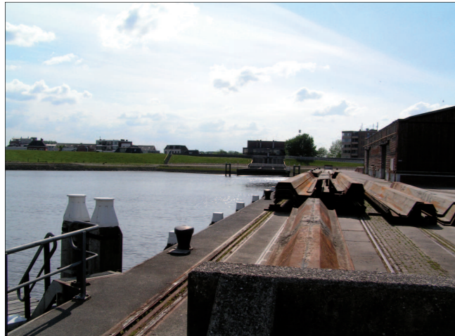
Damsterkade: vacant and dilapidated
