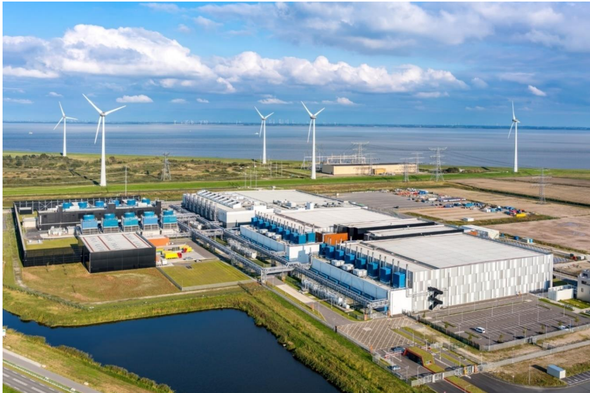
Google data center in Eemshaven, The Netherlands (Google, n.d.).
