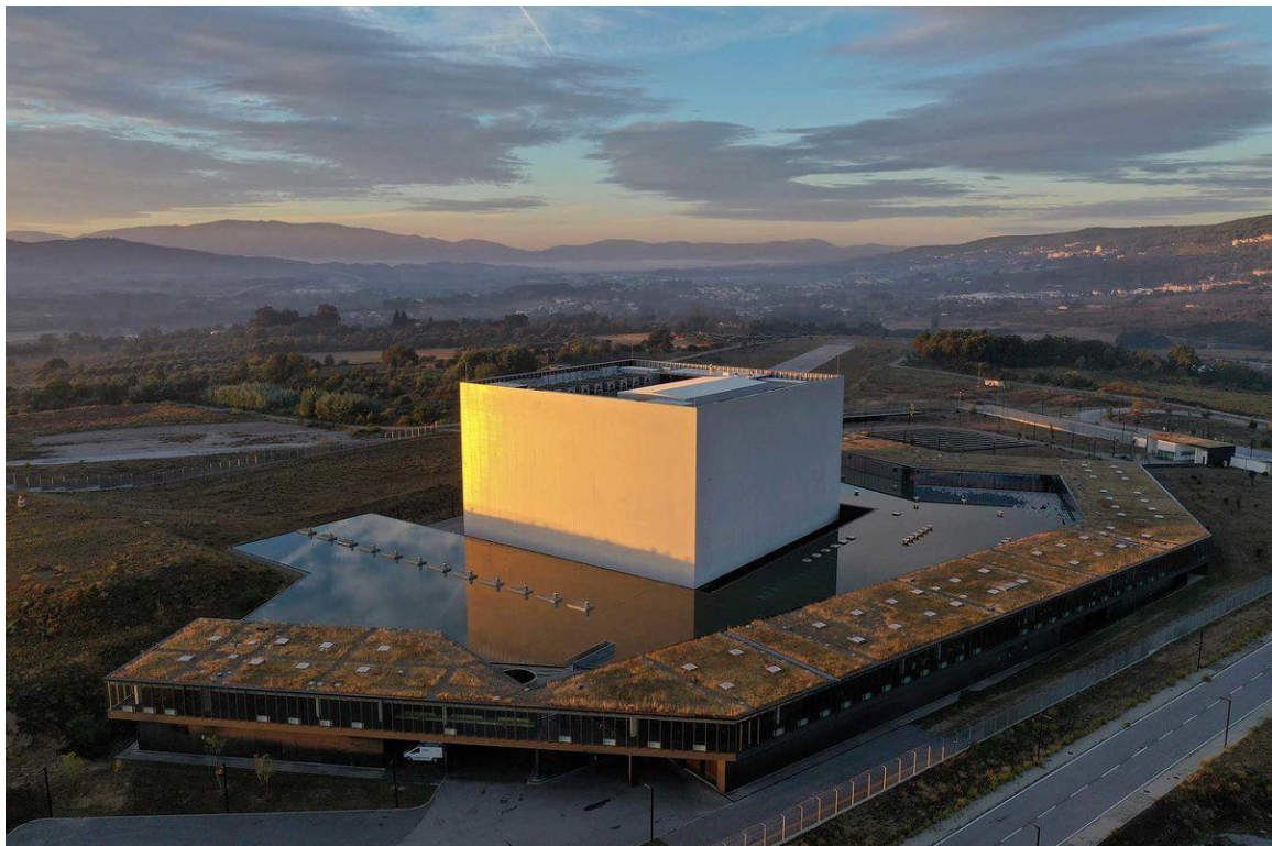
Altice data center in Covilhã, Portugal (Price, 2018).
