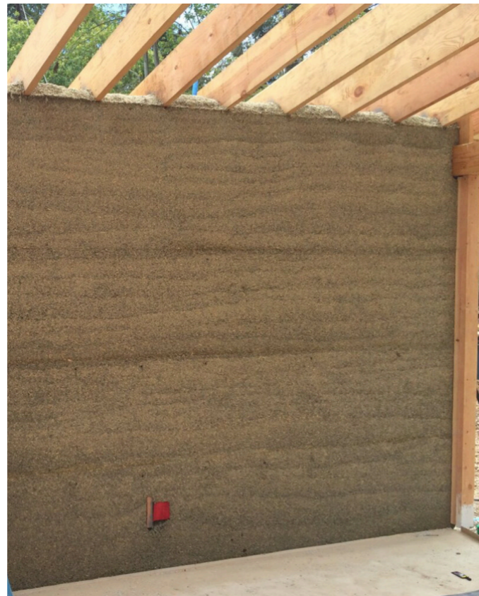
Figure 4.7: Hempcrete wall (Hemp build magazine, 2021)
