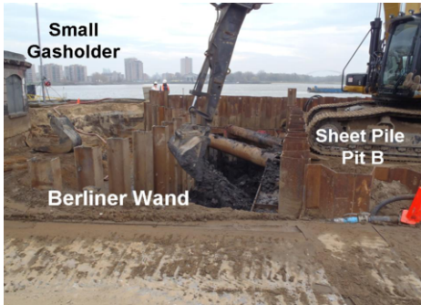
Figure 8. Deep excavation in section E
