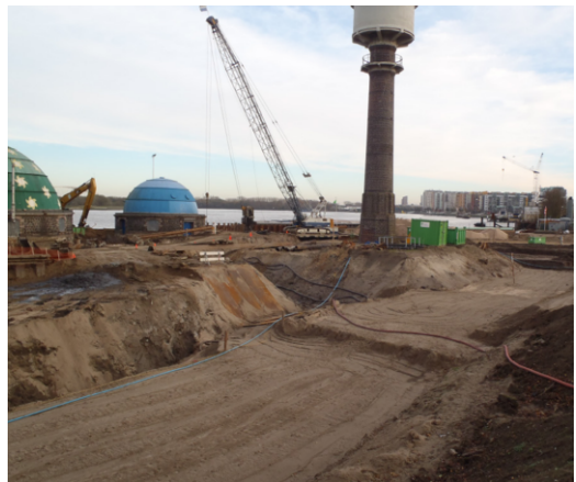
Figure 9. Excavations around water tower
