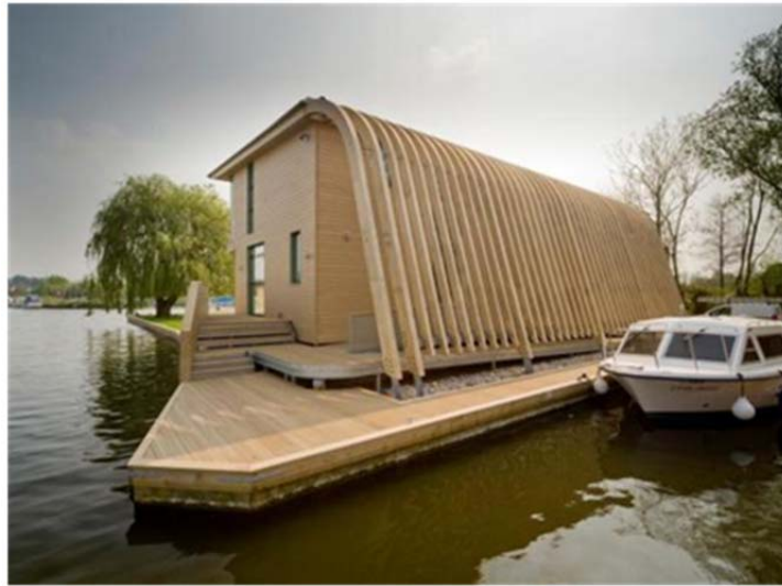
Figure 2: Accoya ® wood used for cladding, decking and structural beams in boathouse in Horning, Norfolk, UK.
